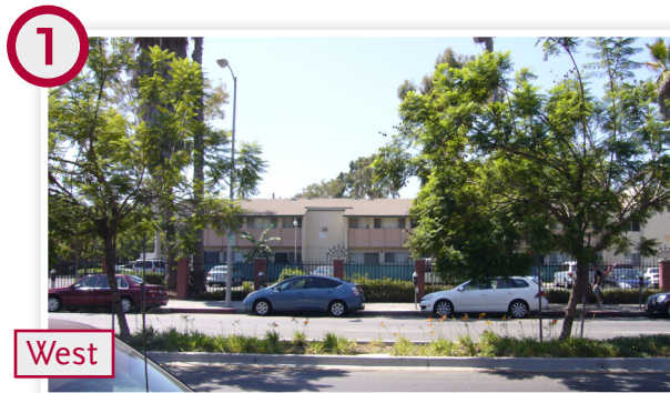
Two-story apartment buildings set back from the street and buffered with fencing and landscaping define the west side of Vermont nearest Jefferson.
